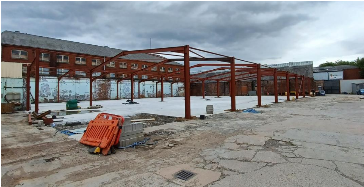
Photo 4: View of partially constructed building
